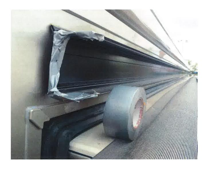
• Tape end of frame and front of cradle to prevent the fabric from snaging on sharp edges.
