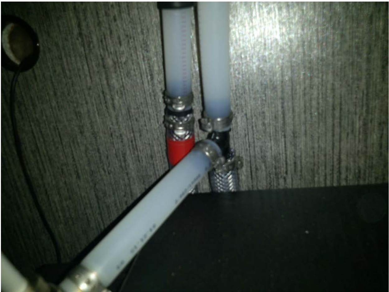
Figure 2 heated hot/ cold water line in kitchen cabinet area
