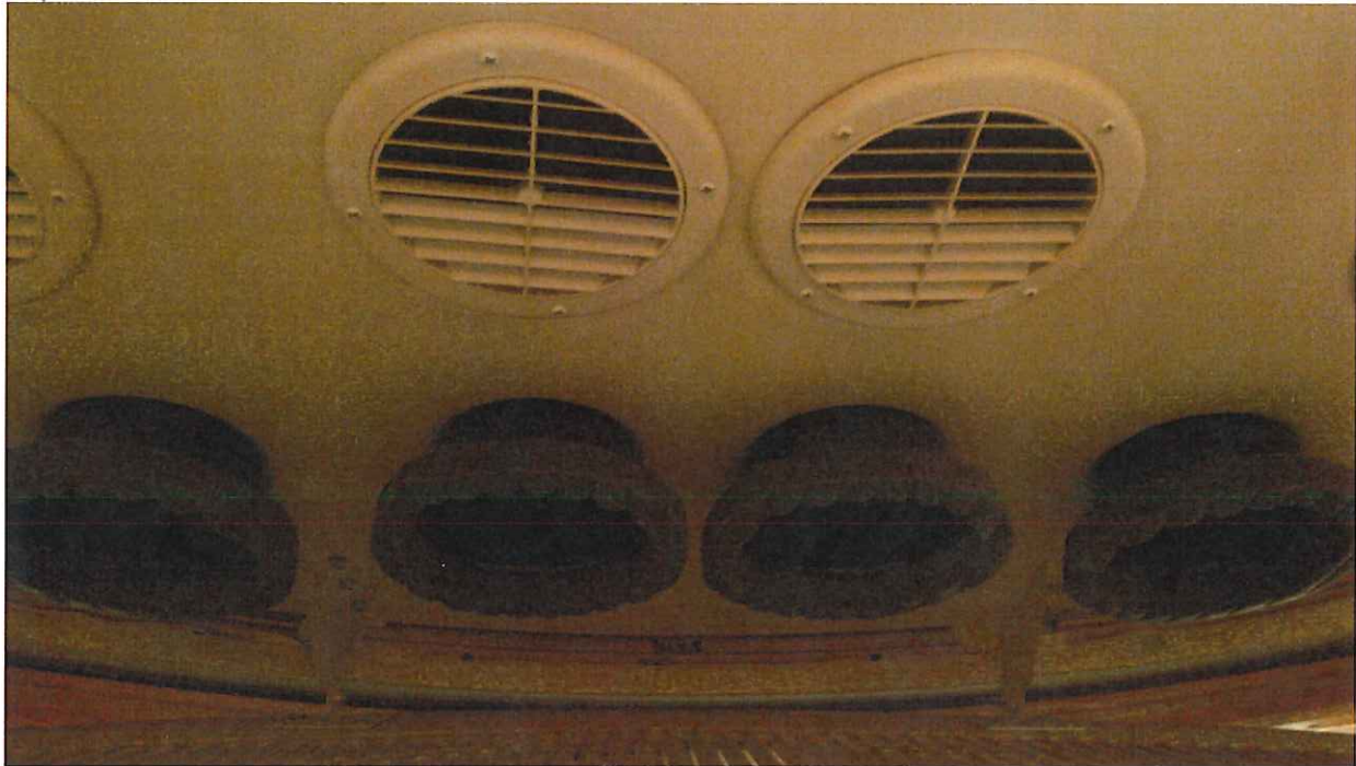
Ceiling feature opened exposing discharge vents
