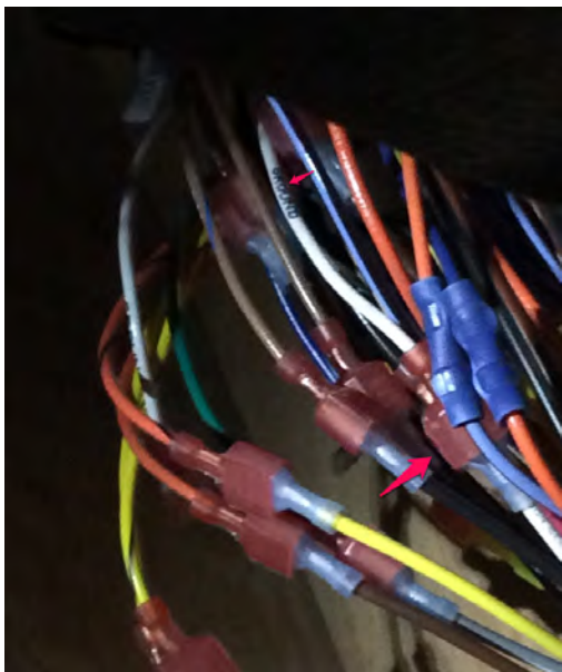
Shade Module Ground Wire
