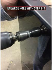
6. Using the drill and a step bit, start drilling the hole for the switch from the painted side of the door. Drill slow to prevent damage to the paint.
