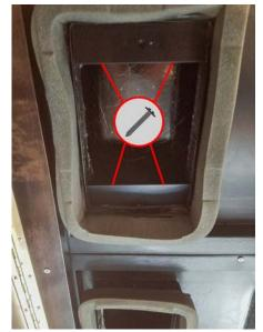
3. Install one angle on each end of the plenum discharge ports. There are three ports under each lattice, so there are 18 ports total.
