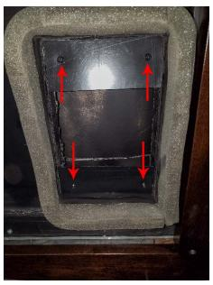
4. Once all angles are installed, install the ABS strips to both angle pieces on the rear port of each plenum. Repeat this procedure at the remaining two rear plenum ports.
