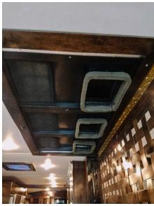
2. Open the lattice panel to access the black plastic air plenum.
