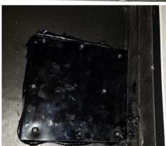
8. Seal the corner, edges, and screw heads using black Sikaflex.
