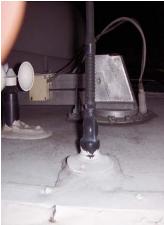
Figure 1 - This shows the roof mounting of a 12" black AM/FM radio antenna.
