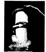
Insert PVC pipe into WASTE ONLY fitting with twisting motion and hold for 30 seconds.
